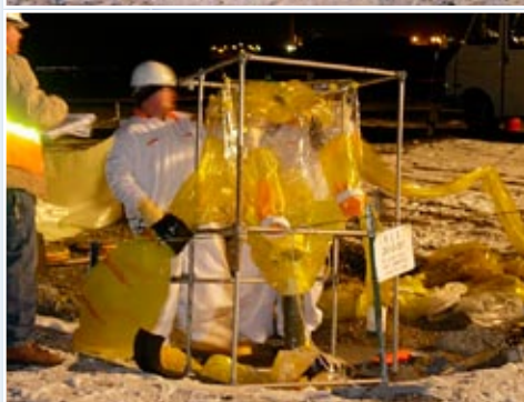
Carefully using measures to control contamination, workers insert a camera through a riser (all photos) in Tank U-361.
